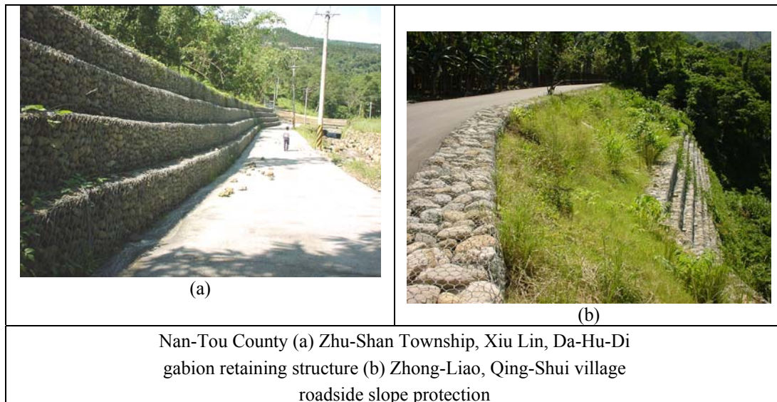
Fig. 1 Gabion structures for retaining wall and slope protection in Taiwan
