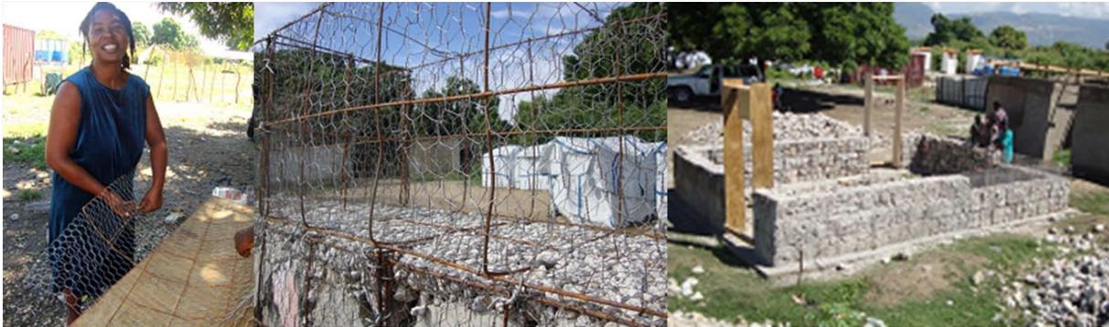
*Figure 1: The construction, placement and layout of gabions*
